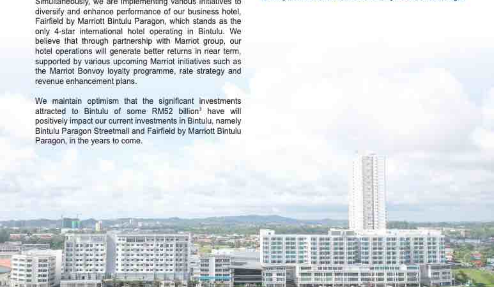
Aerial perspective of Bintulu Paragon which includes Fairfield by Marriott Bintulu Paragon.
