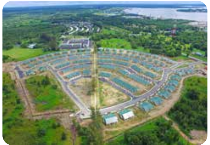
Tanjung Manis Housing project completed in March 2019
