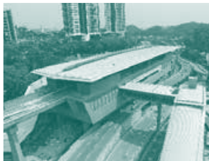
Klang Valley Mass Rapid Transit (KVMRT) Line 1 (Pusat Bandar Damansara station)
