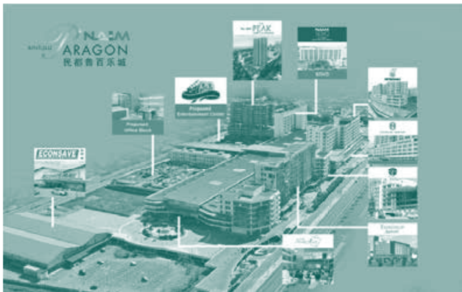
Naim Bintulu Paragon Integrated Development, Phase 1
