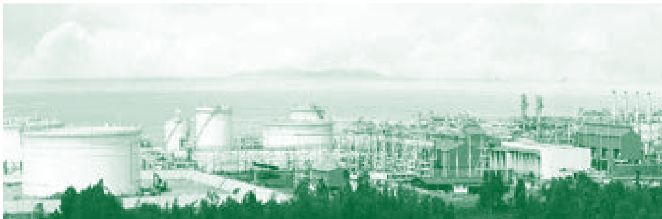
Sabah Oil & Gas Terminal (SOGT) project, Sabah
