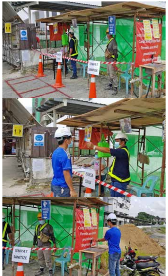
Entrance to project site
