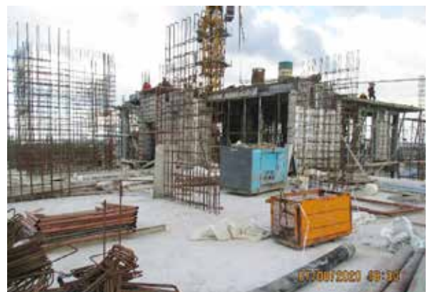
Formwork at Sapphire
