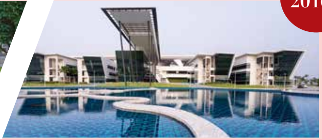
Adjudged the winner of the QLASSIC Excellence Awards 2016 (for building construction quality) in the Non-Residential (Large) category for our JV project with Hock Peng Furniture & General Contractor Sdn Bhd, the University College of Technology Sarawak (UCTS) (Phase 2, Stage 1) in Sibul
