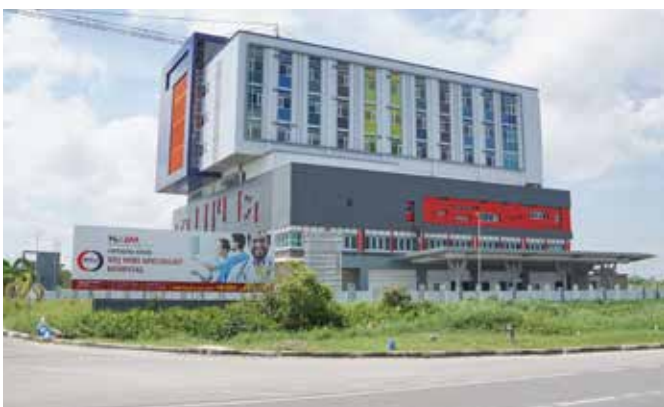
Recent site progress photo of KPJ Miri Specialist Hospital
