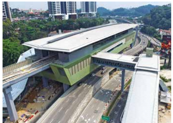
One of the elevated MRT stations built by Naim in Peninsular Malaysia
