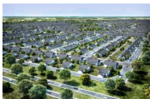
On-going projects - housing construction
