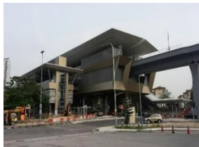
Substantially completed project - MRT stations
