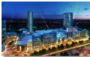
On-going project - Bintulu Paragon
