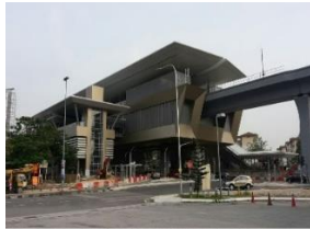
Substantially completed project - MRT stations
