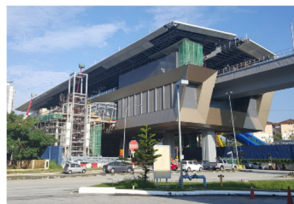
MRT stations under construction
