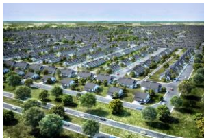
On-going projects - housing construction
