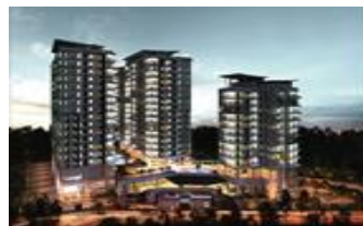
On-going project - Kuching Paragon
