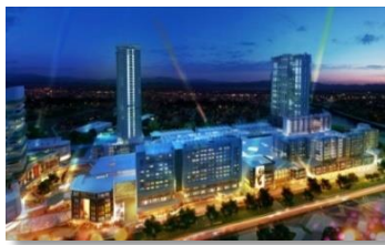
On-going project - Bintulu Paragon
