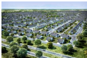
On-going projects- housing construction
