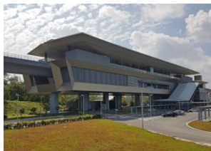
Completed project - MRT stations
