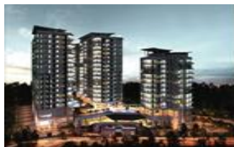
On-going project - Kuching Paragon
