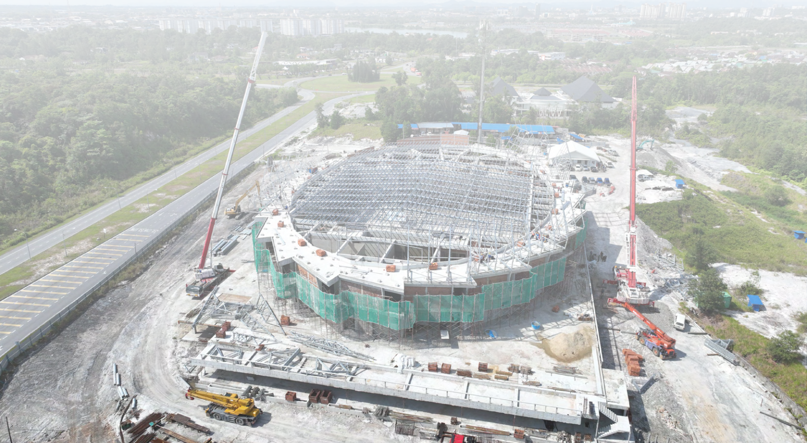
Aerial shot of Wisma Melayu construction site in early 2024.
