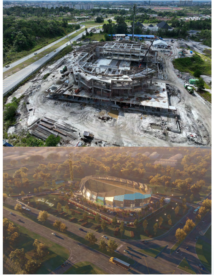
Construction of Wisma Melayu as at November 2023 (Top) and Artist Impression of Wisma Melayu (bottom)
